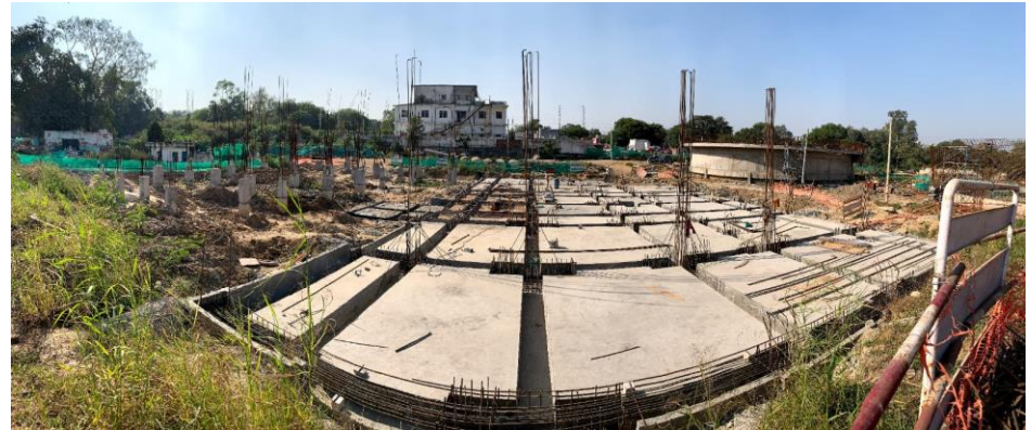
Construction work is going on. The above : Ozone Contact Tank The left : Ozone Building
